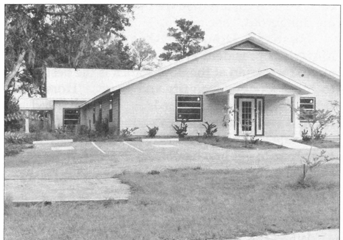
The attractive activities building was more than 50 percent complete when the merger took place. It faces the pond and is approached through a paved road.
