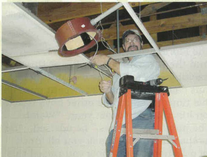
This ceiling is receiving some lighting upgrades from Jim Swanner.
