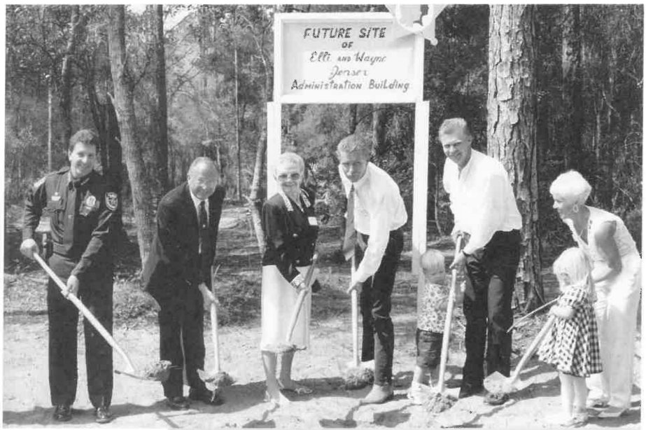
Volusia County Sheriff Bob Vogel joined Wayne and Elli Jensen and their family as they broke ground for the much needed Wayne and Elli Jensen Administration Building.
