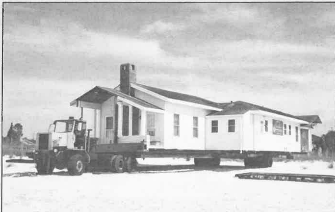
The Tralins building was moved by barge and trailer from Clearwater Beach to Caruth Camp, a distance of approximately 90 miles.
