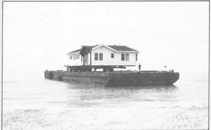
The Tralins building was moved by barge and trailer from Clearwater Beach to Caruth Camp, a distance of approximately 90 miles.
