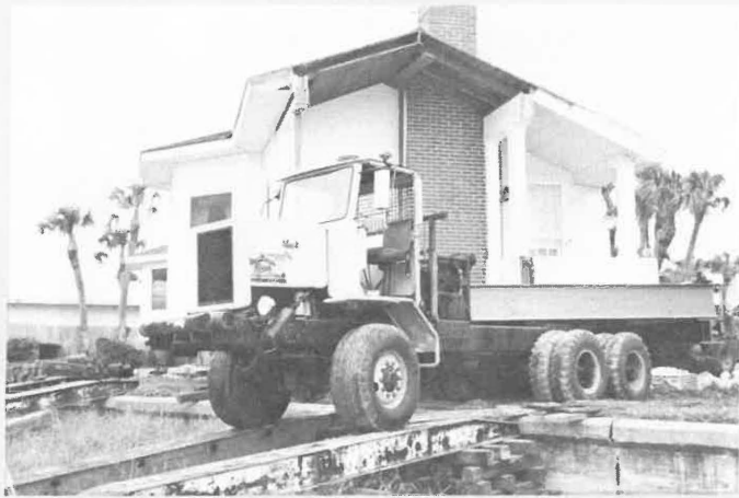
Crossing a seawall was no problem at all.
