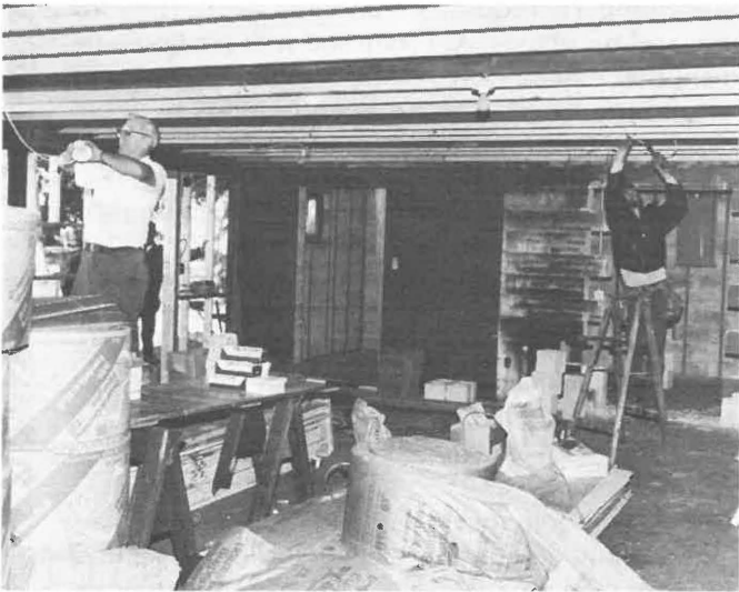
Rewiring, winterizing and other improvements began before the end of 1985.
