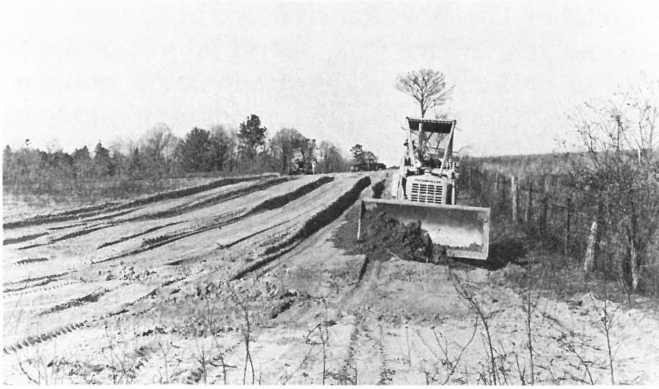
Construction of Boys Ranch roads began in 1957.
