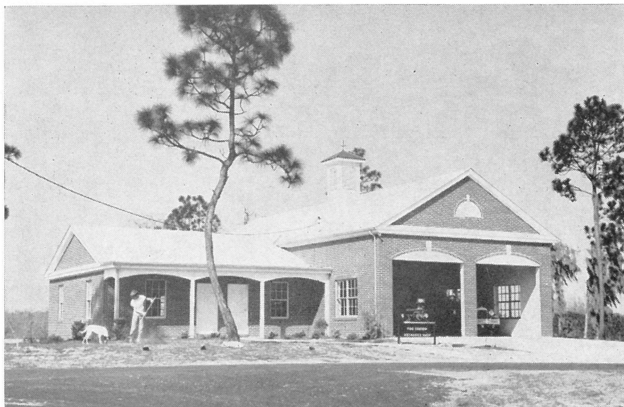
The $35,000 Fire House and Repair Shop built by the Florida State Firemen's Association is already in use although the interior is not completed.
