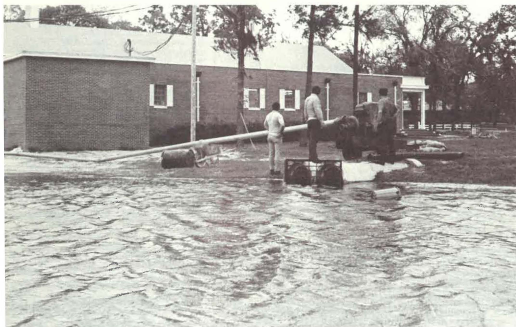
Flood waters backing up through large storm sewers created a lake that threatened to inundate the cafetorium. Emergency pumping failed to stop the rising water; but sandbags dropped through a manhole temporarily plugged the sewer line and solved the problem.
