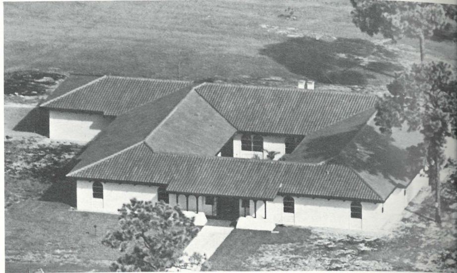
Aerial view of Pinellas Sunshine Villa by Selbypic, Inc., of Tampa.
